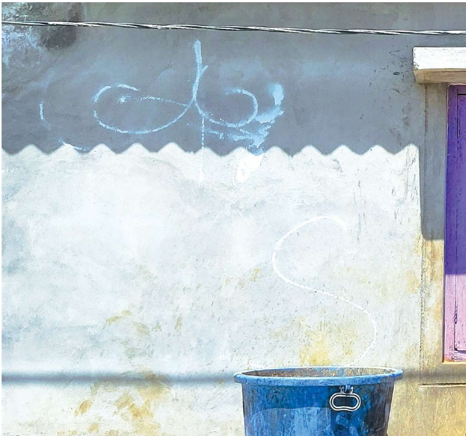
Hanging through the cracks
